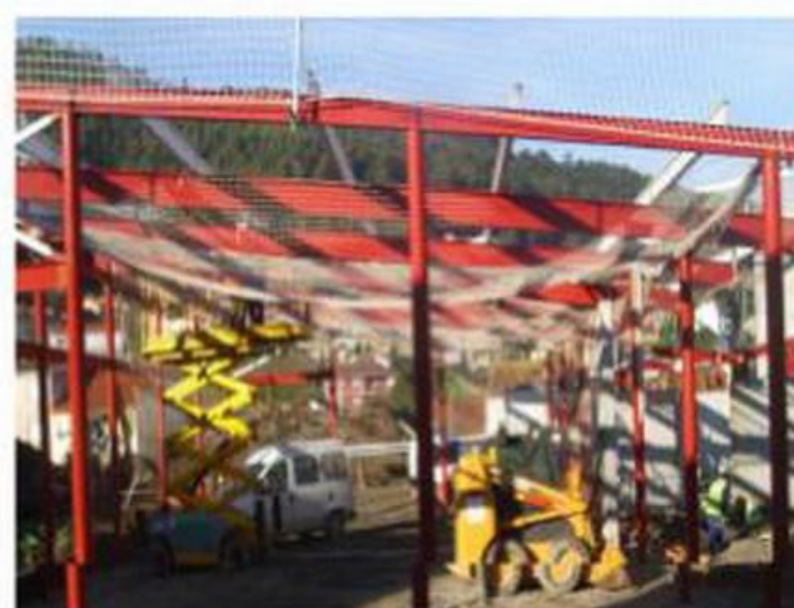
As obras do novo pavillón
